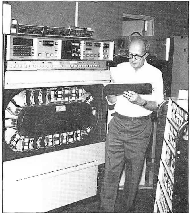
Two TCR-100A "cart" machines handle commercial blocks—about 600 air functions daily.
