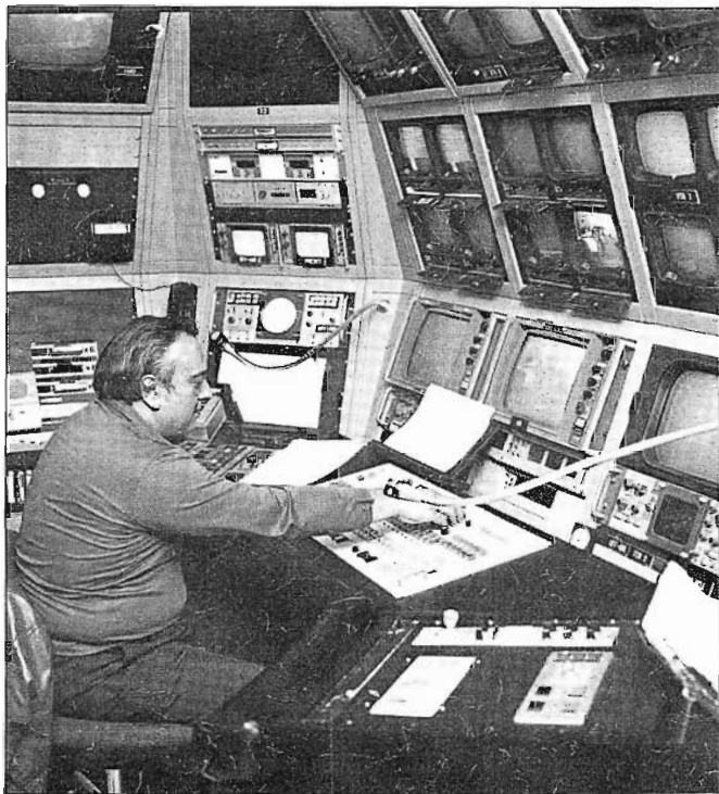
Master Control for TV-38 features a "cockpit" design, with floor-to-ceiling glass, and is configured for operator comfort and efficiency.
